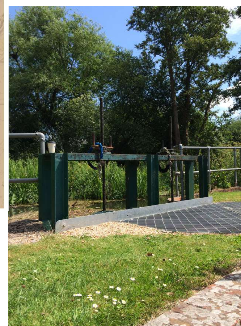
The volume of water flowing into Romsey is now controlled via a sluice. Excess water is diverted into the Horsehead Ditch.
